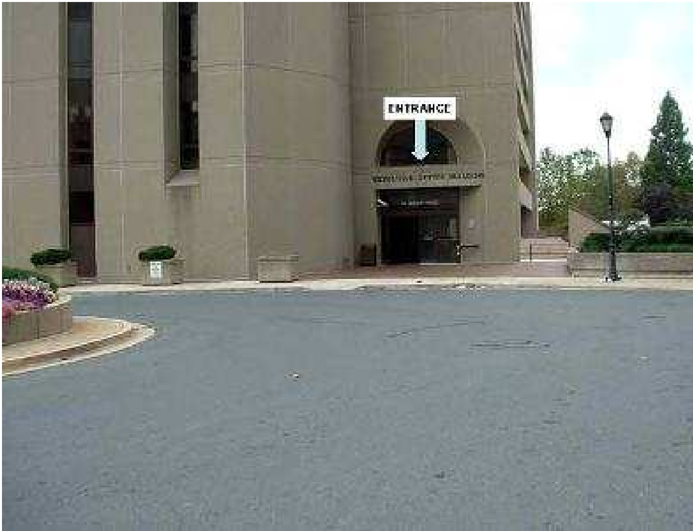
Executive Office Building 101 Monroe Street Rockville, MD 20850
